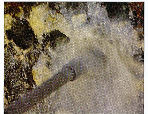
HydroDrilling a Sulfur Recovery Unit
