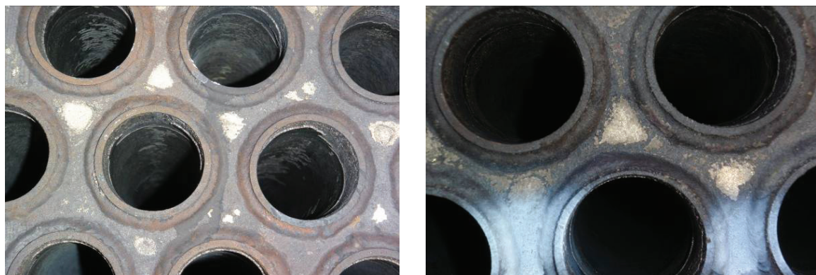
Figure 8. Tube internals after cleaning with NitroLance
