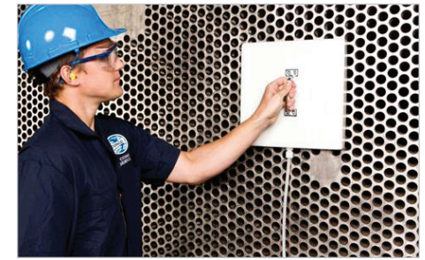
Figure 4. Technician delivering tracer gas through a plenum.
