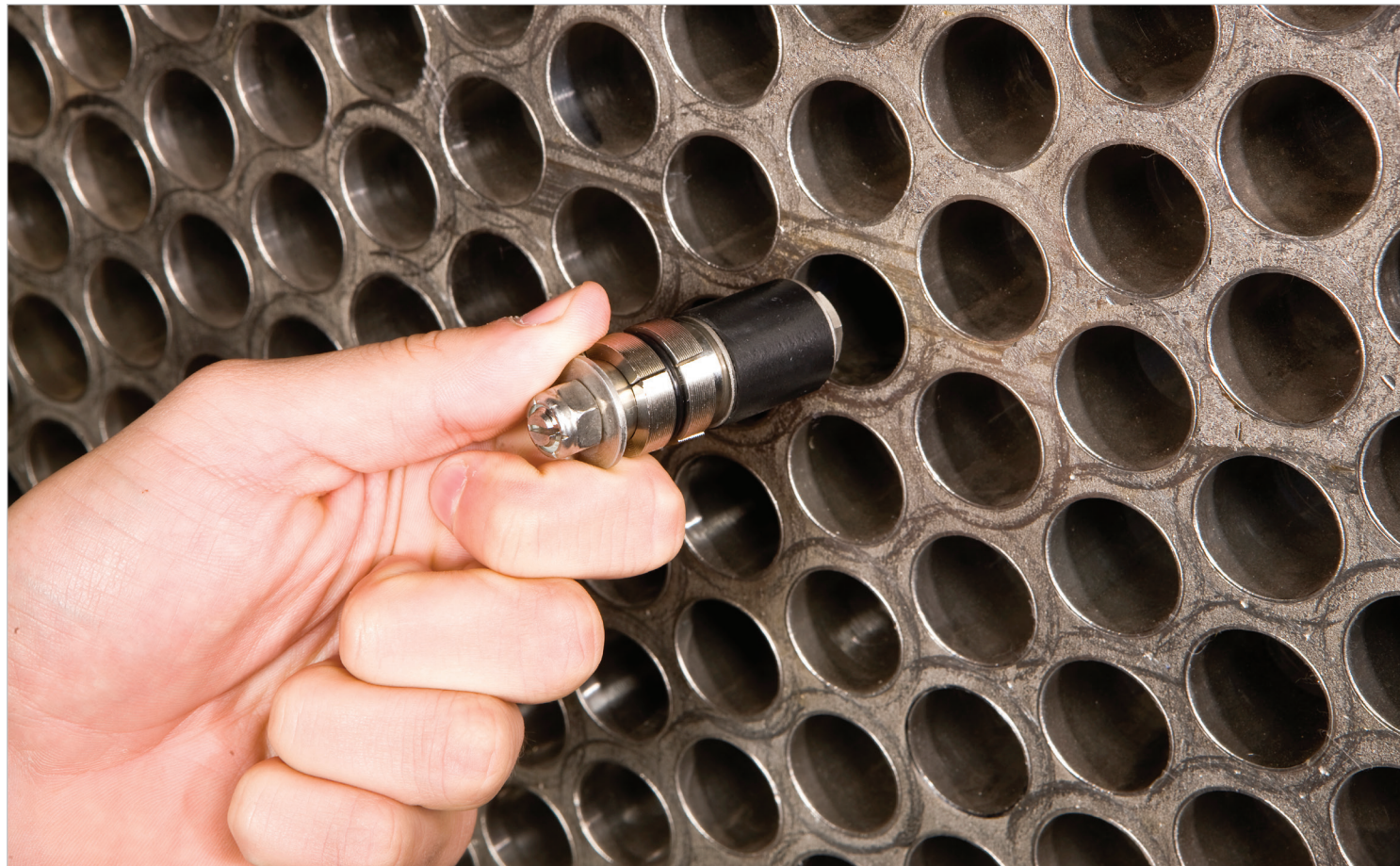
Figure 5. Proper installation of tube plug.
