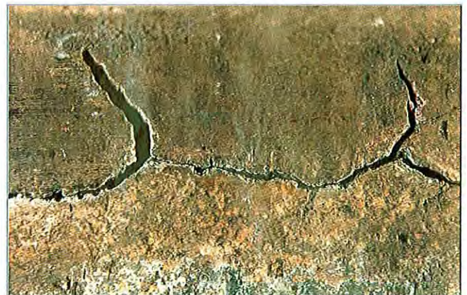
Figure 9: Stress corrosion cracking in admiralty brass tube due to carryover of sulfur dioxide, in sulfite-treated boiler. Magnification 4x.
