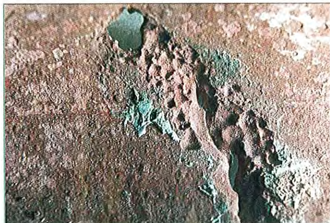
Figure 11: Erosion-corrosion failure in 90-10 copper-nickel tube, due to accelerated local flow around an object lodged in the tube. Magnification 4x.
