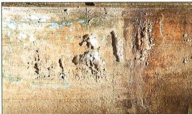
Figure 10: Inlet-end erosion-corrosion in admiralty brass tube. Magnification 3x.
